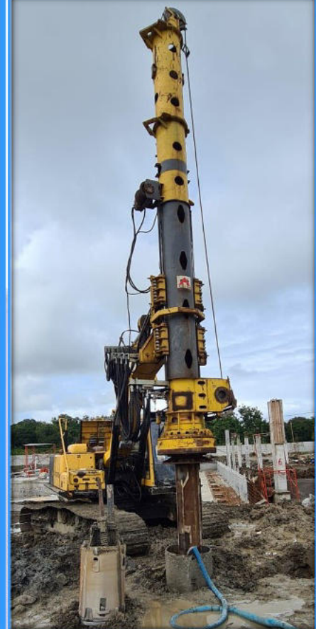
Drilling Machine (Borepile) VOLVO E210
